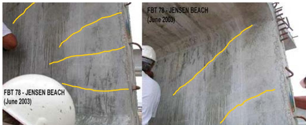
**Figure 1-1: Bursting and Spalling Cracks in Florida Bulb Tees: Jensen Beach**
