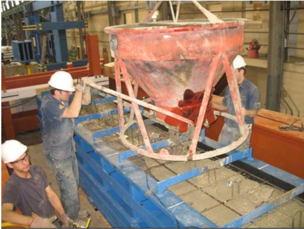
*Figure 3-46: Concrete placement using a 1 cy hopper*
