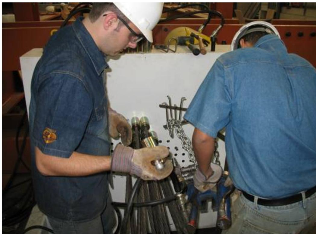
*Figure 3-40: Individual strand stressing with mono-strand stressing jack*
